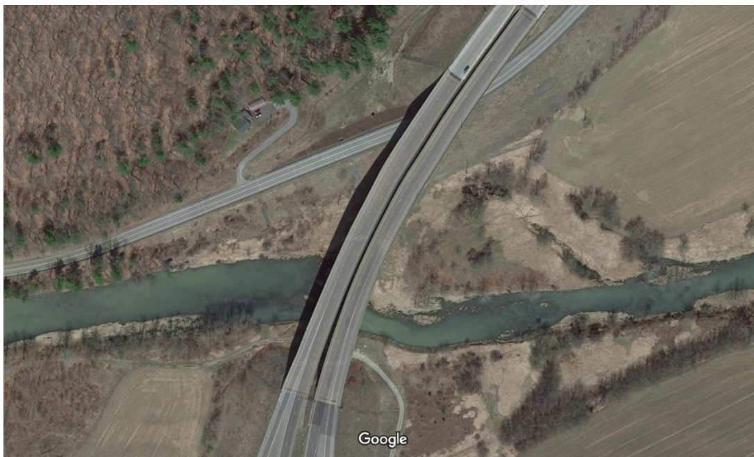
Figure 3-5: Aerial View of Selected Horizontally Curved Bridge (Google Maps n.d.)
